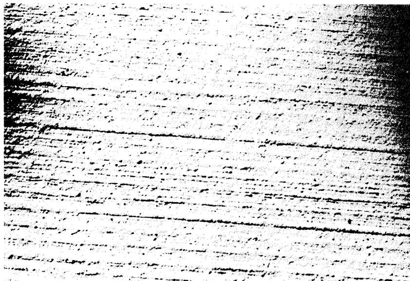
Fig. 2-6. Test Section F-1: Transverse broom finish (as constructed)
