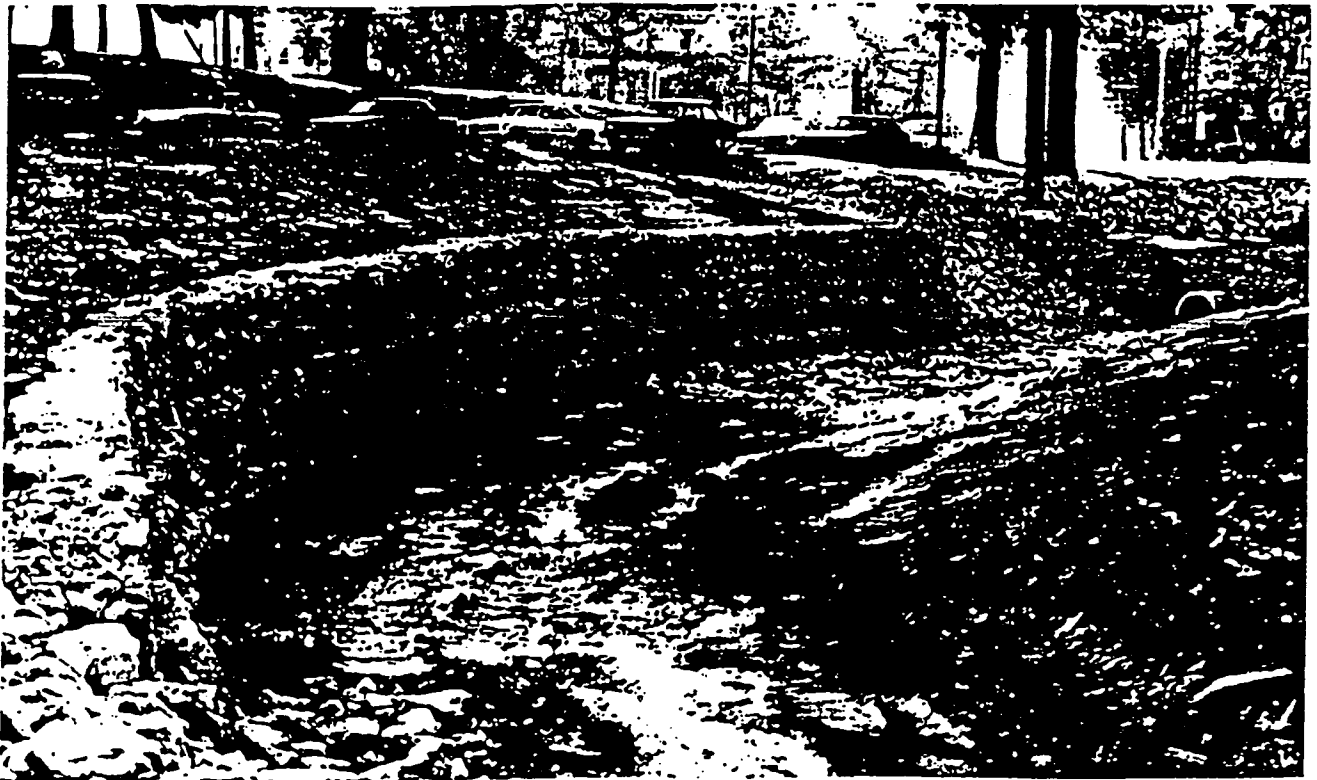
Structural streambank stabilization such as gabions and riprap is necessary where stream velocities are high and side slopes are steep.
