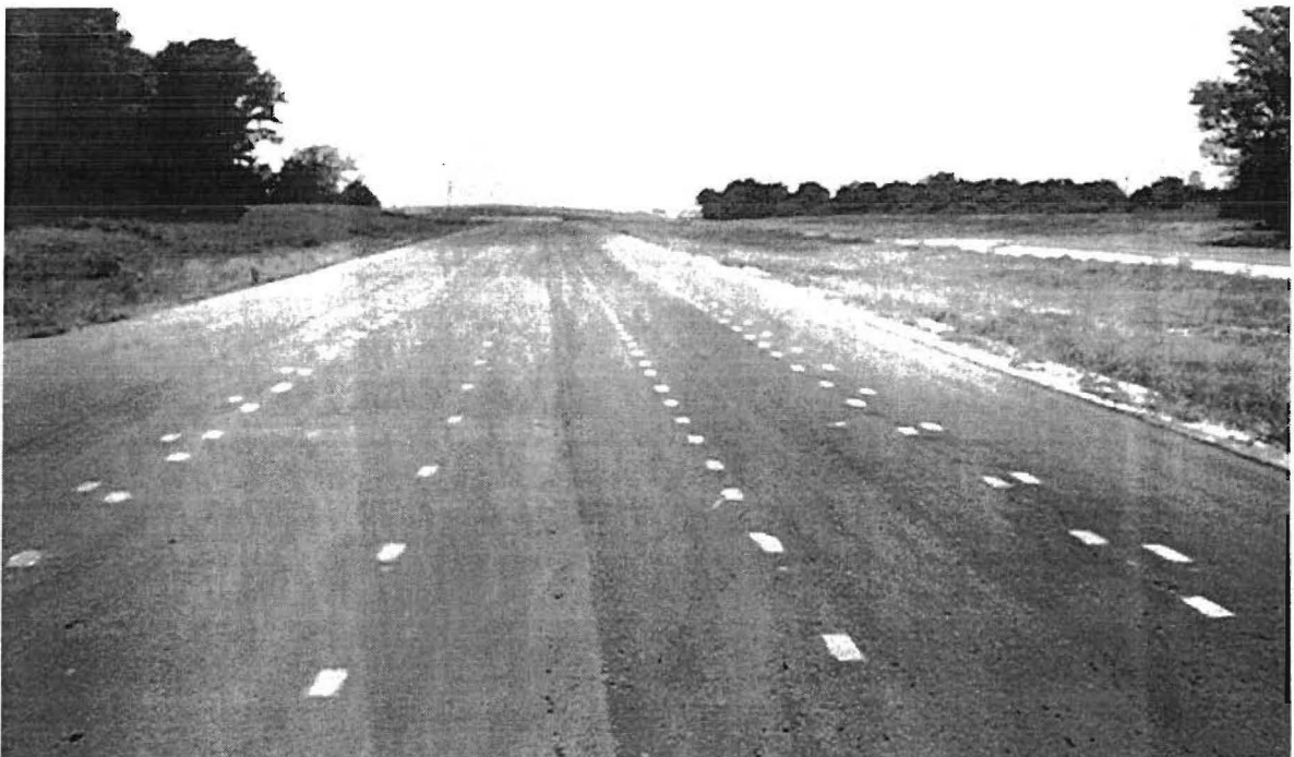
Figure 3. Sites SH47A (left) and SH47B (right) Located on Adjacent Lanes of SH47.
