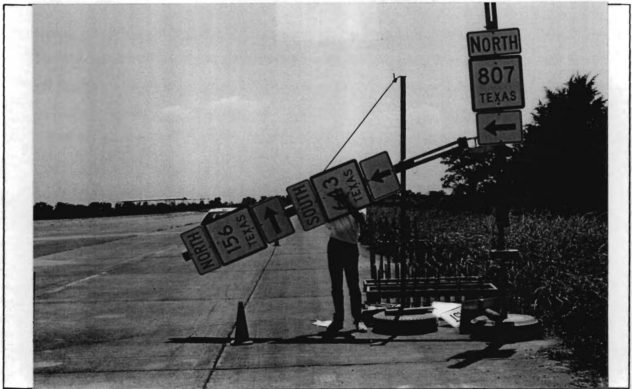
Figure IV-1. Typical Sign Installation
