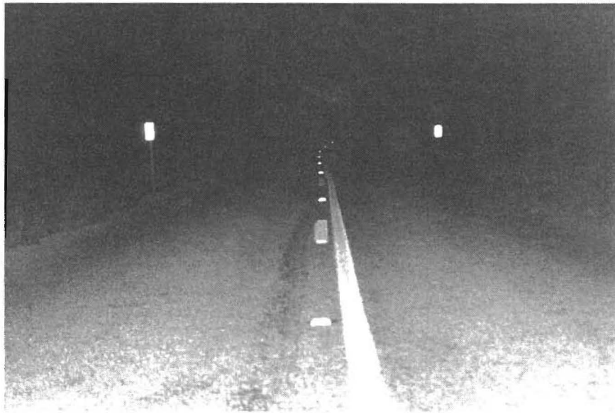
FIGURE 2-1. Type OM-2 Object Markers at Culvert Ends
