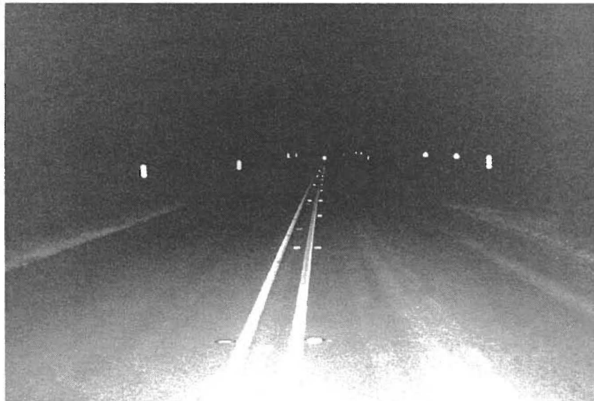
FIGURE 2-3. Type OM-2 Object Markers and Post-Mounted Delineators at Bridge Ends
