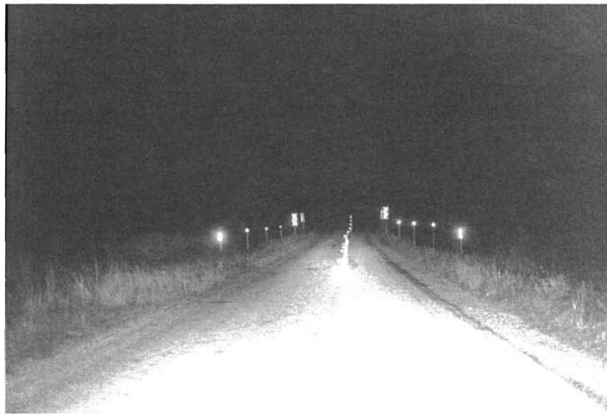
FIGURE 2-4. Type OM-3L and OM-3R Object Markers and Post-Mounted Delineators at Bridge Ends
