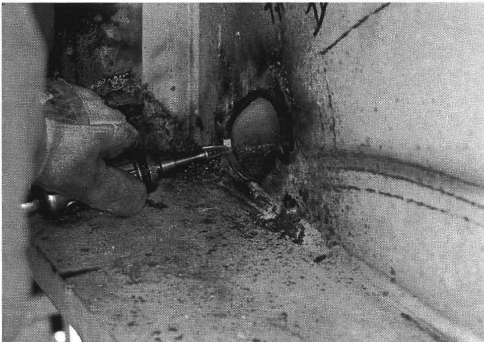
Figure 2-11: Grinding of hole to a smooth surface.
