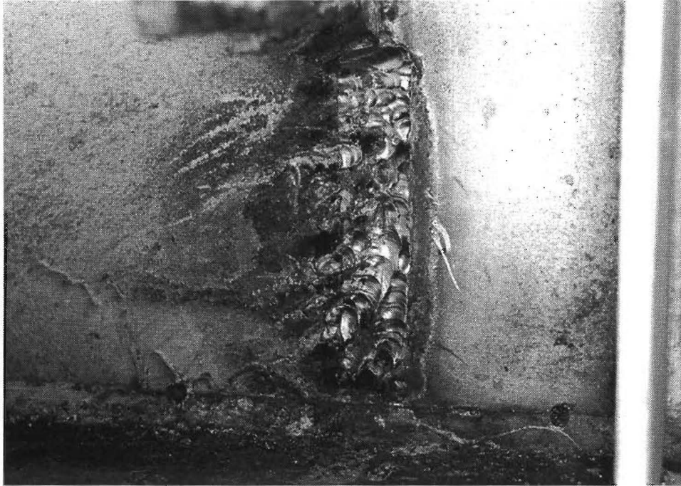
Figure 2-2: Web plate after removal of connection plate end by air-arc gouging.
