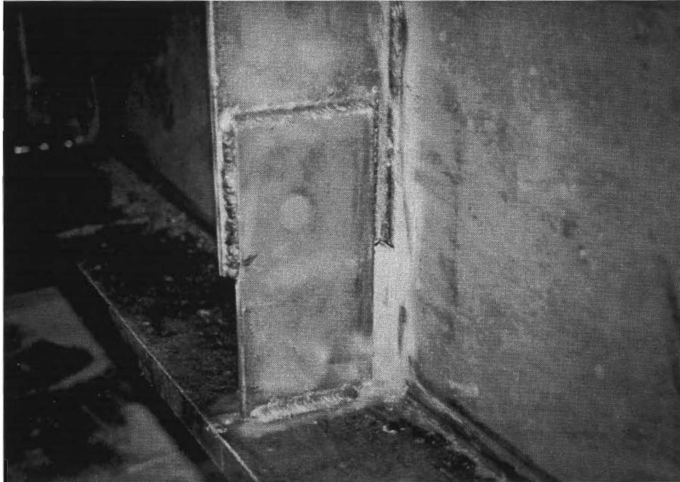
Figure 3-34: Tight-fit retrofit using welded clips.
