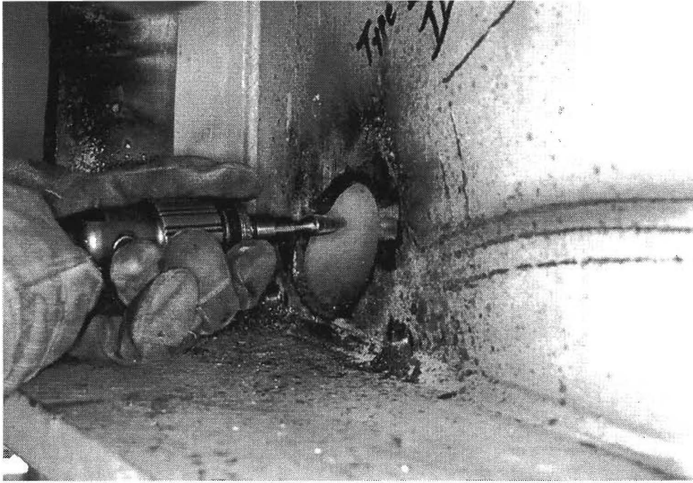
Figure 5-12: View of die grinder used to finish holes.
