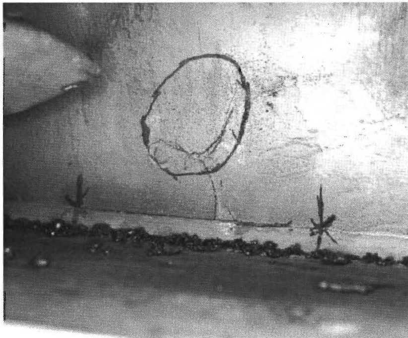
Figure 5-10: View of outlined hole for flame-cutting.
