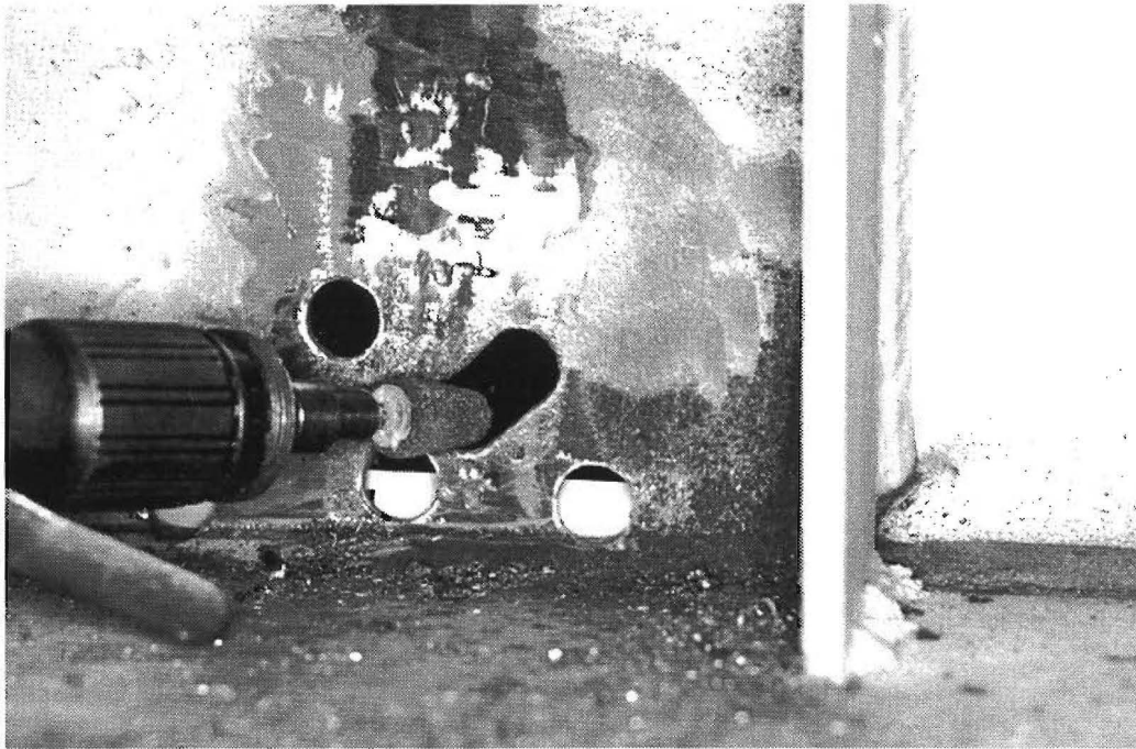
Figure 2-20: Repaired web section after hole-slotted.
