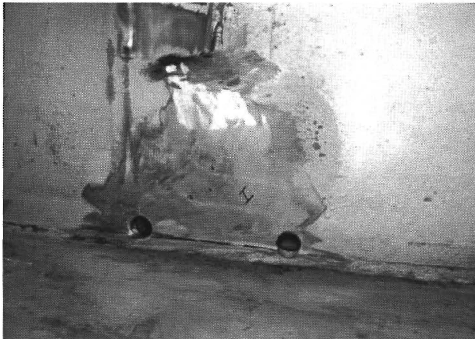
Figure 2-21: View of completed Type I repair procedure.
