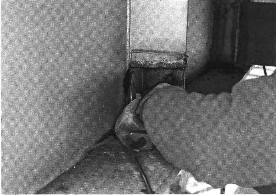
Figure 2-3: Grinding to remove remaining web material and connection plate.
