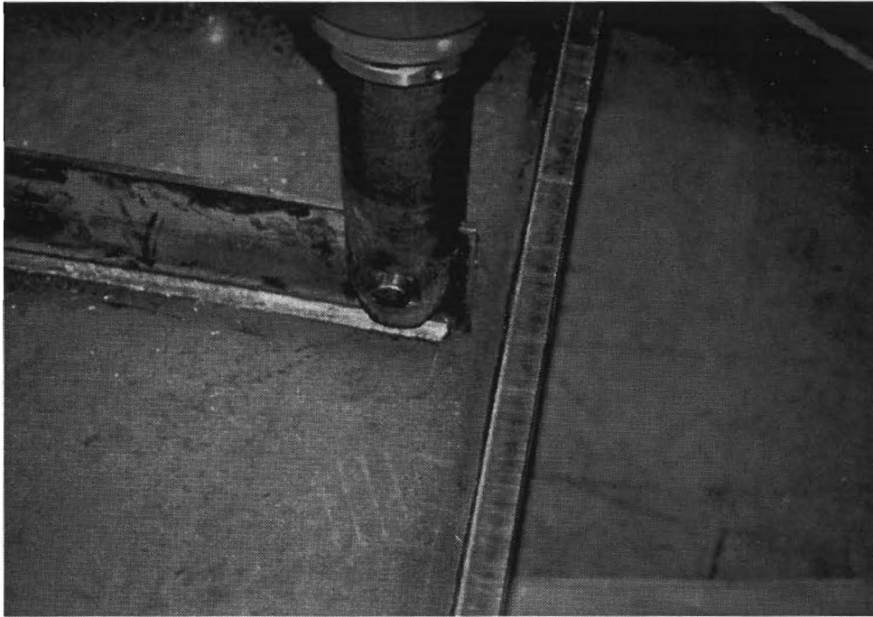
Figure 3-8: Pre-cracking of Girder 2.
