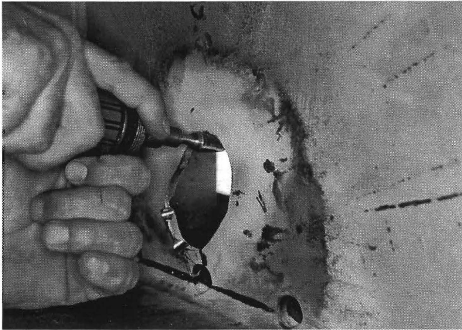
Figure 2-14: Removal of remaining cracks with grinder.
