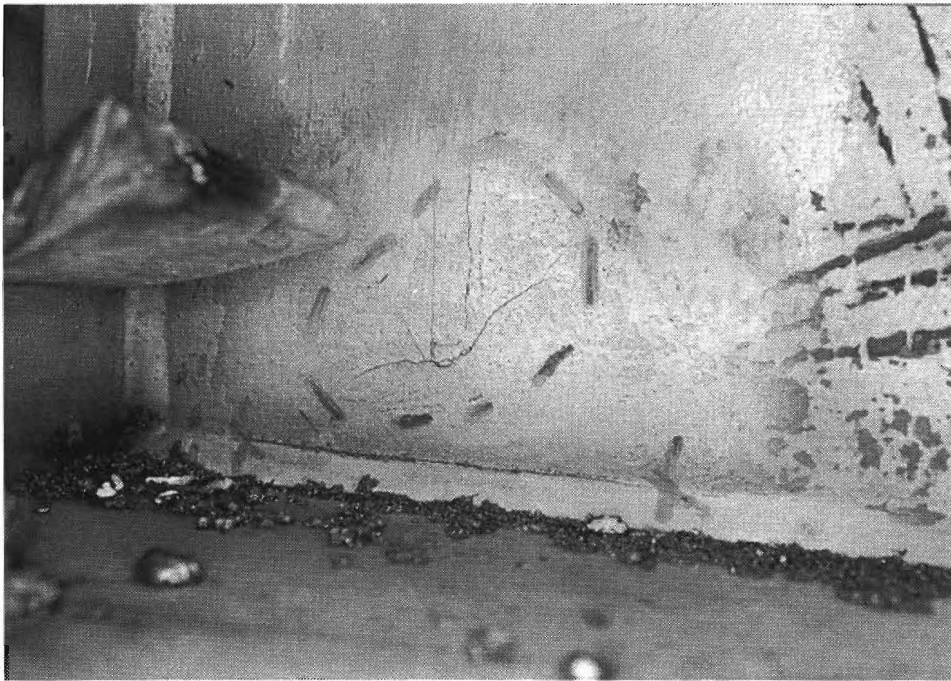
Figure 2-9: Location and marking of the cracked area.
