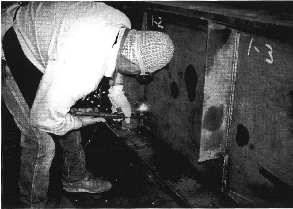
Figure 3-21: Shortening of stiffeners by flame-cutting.
