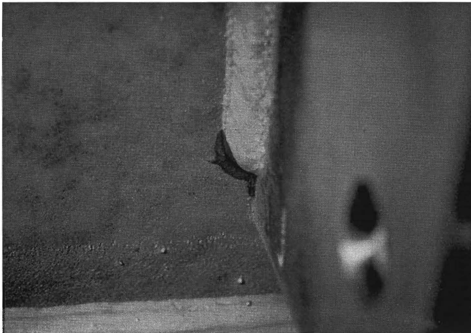
Figure 3-16: Examination of crack using dye penetrant.
