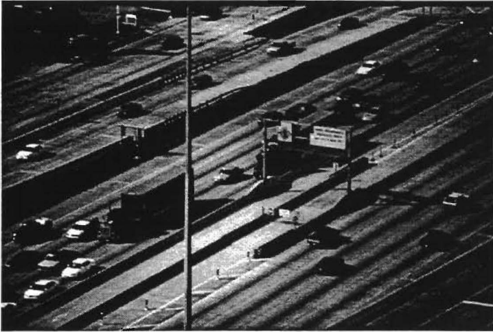
Figure 41. Slip Ramp for HOV Lane Access/Egress on Katy Freeway
