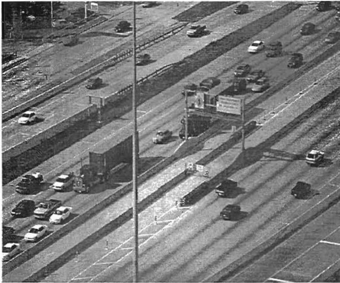
Figure 4. Slip Ramp for HOV Lane Access/Egress on Katy Freeway
