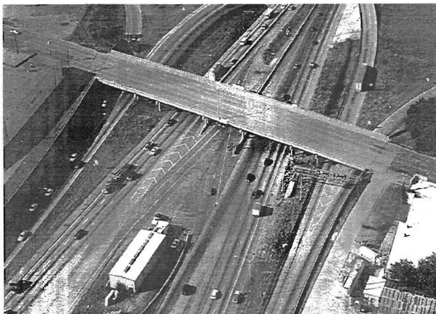
Figure 9. Example of Access Point of East R.L. Thornton HOV Lane
