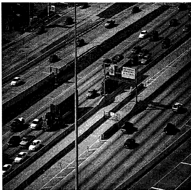
Figure 6. Slip Ramp for HOV Lane Access/Egress on Katy Freeway
