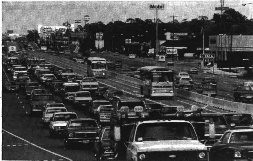
Figure 5. HOV Lane in Median of Katy Freeway
