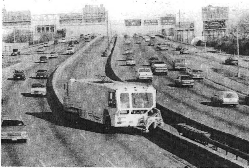
Figure 9. Machine Used to Shift the Moveable Concrete Barrier on East R.L. Thornton
