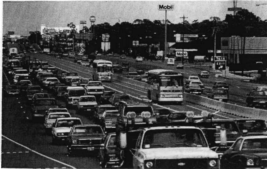
Figure 5. HOV Lane in Median of Katy Freeway
