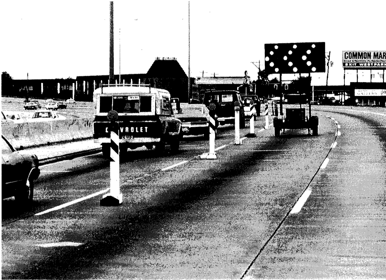
Figure 28. Lane Closure Traffic Control
