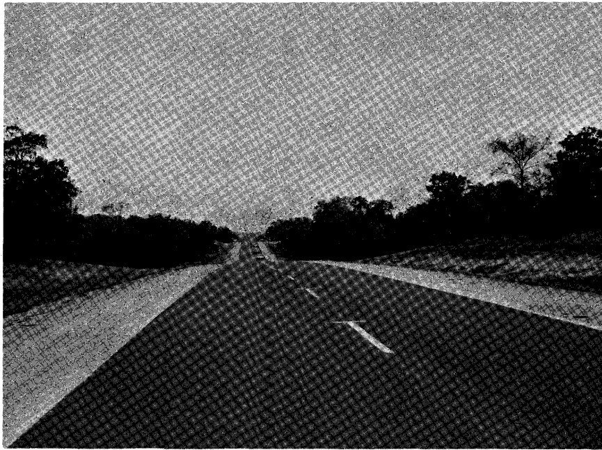
(c) View from beginning of Site P-2 passing zone looking back through impeding zone
