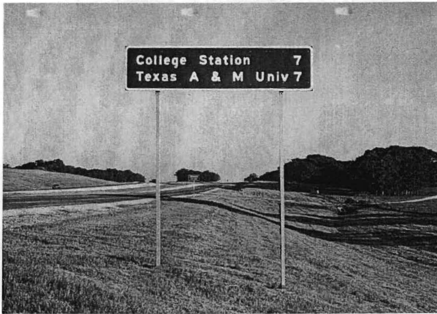
FIG. 1. Typical Roadside Sign Installation
