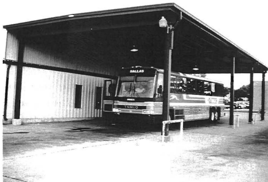
Figure 35. Picture of Bus Station with Shelter.
