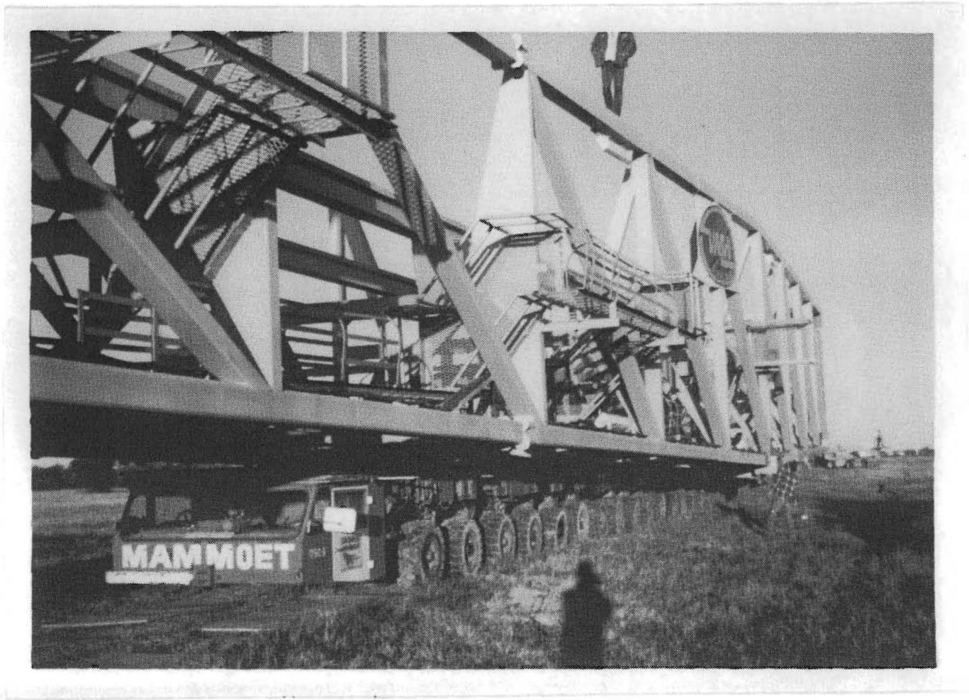
Figure 2. Photograph of the tower load moved at Victoria.
