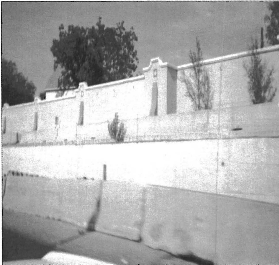
Figure 21. Traffic Side of Sound Wall, U.S. 75 in Dallas (68 dBA).
