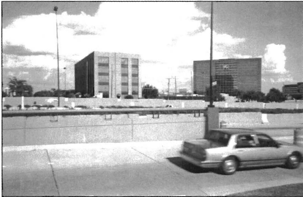
Figure 19. Concrete Noise Barriers and Slightly Depressed Main Lanes.
