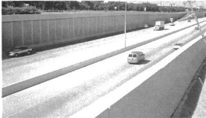
Figure 15. Depressed Section of U.S. 281 in San Antonio.
