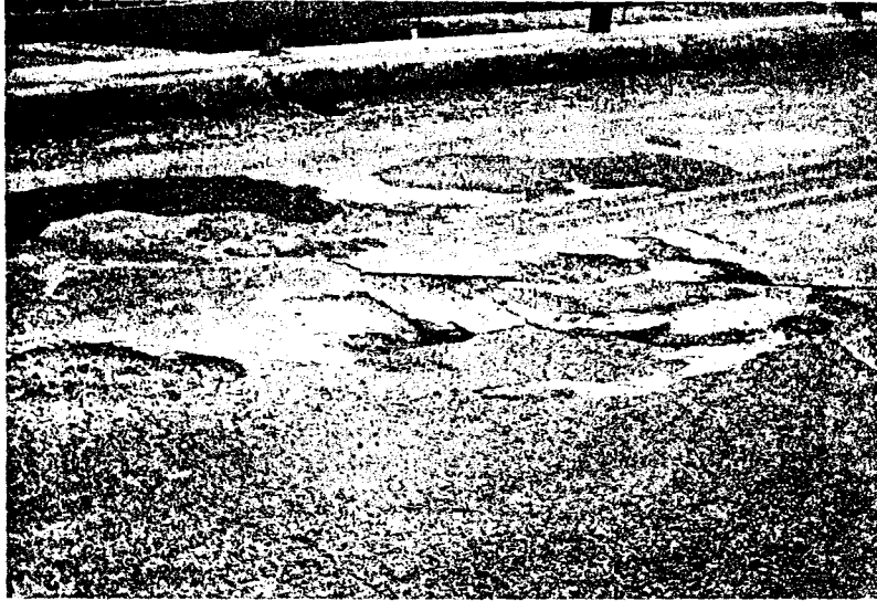
FIGURE 1: A typical delaminated area of a bridge deck in the last stages of deterioration.
