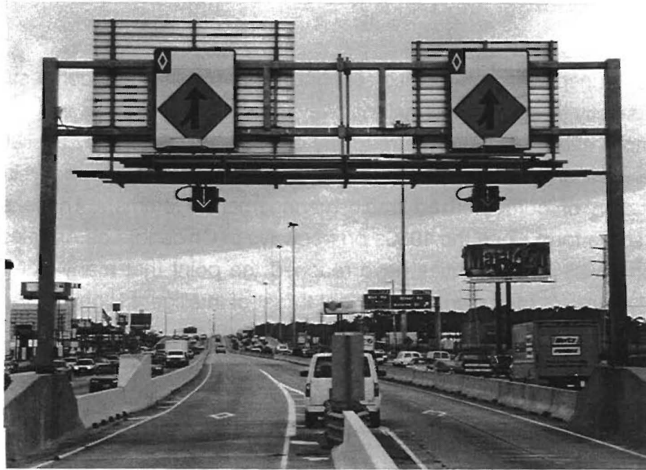
Figure 1-1. Lane Control Signals on High-Occupancy Reversible Lanes in Houston.
