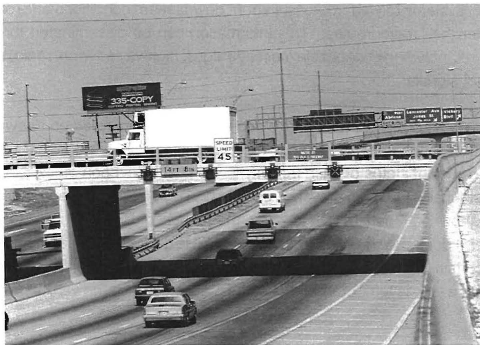
Figure 1-2. Freeway Lane Control Signals on I-35W in Ft. Worth.
