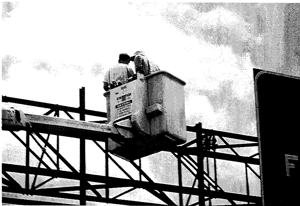
Figure 22. Installation of Video Equipment on Sign Structure.
