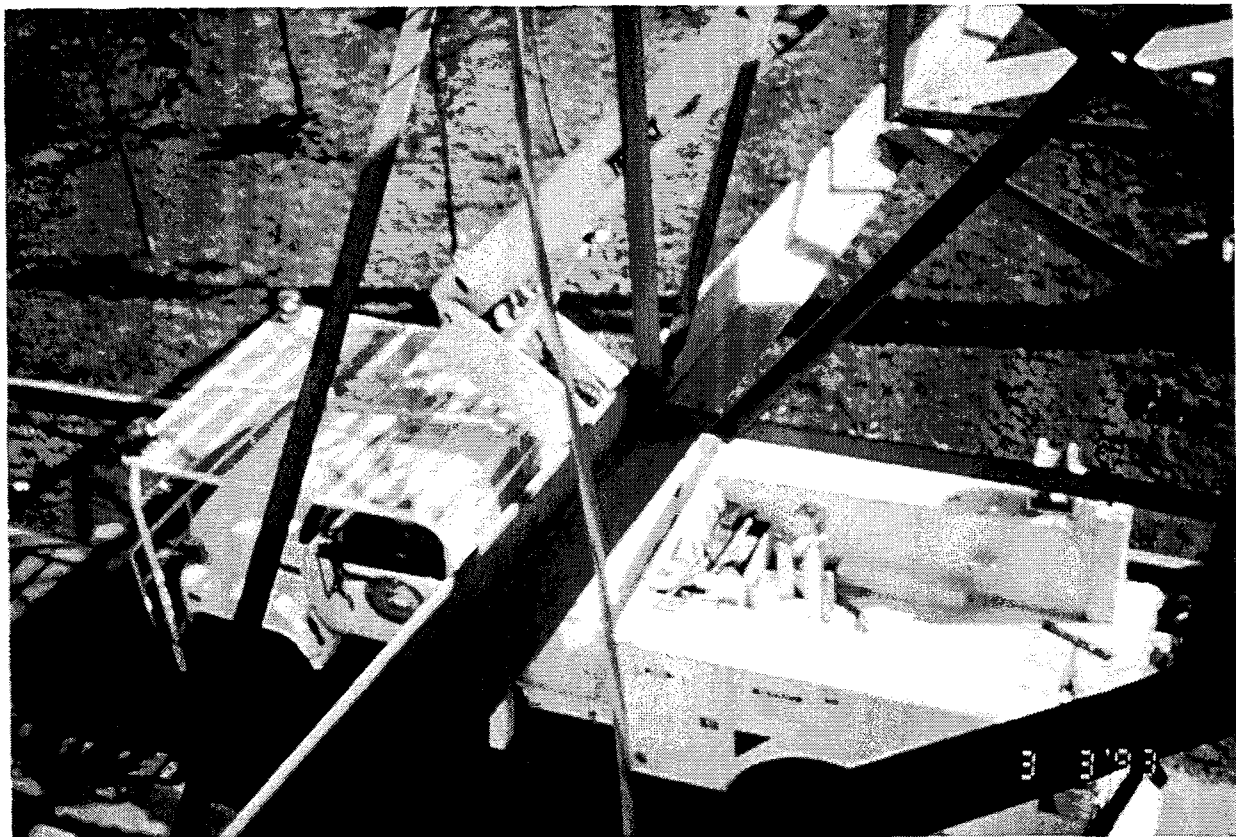
Figure 21. Bucket Truck Used to Install Video Equipment.
