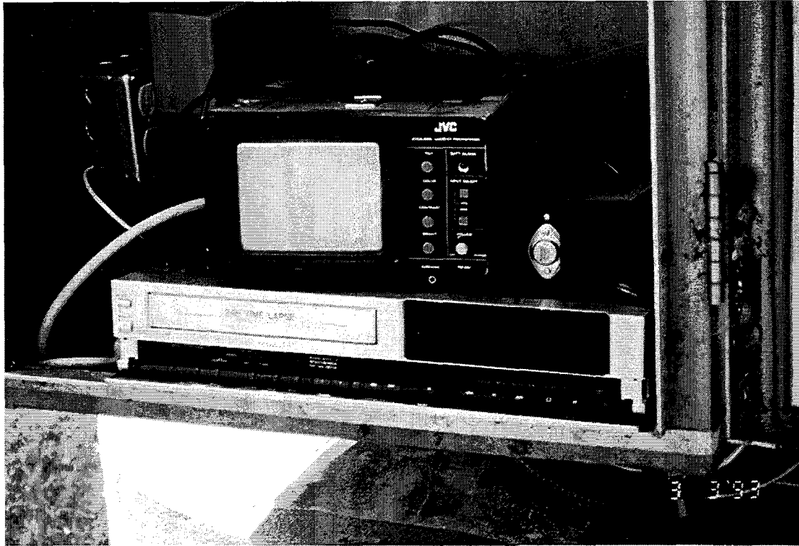
Figure 24. VCR in Controller Cabinet.
