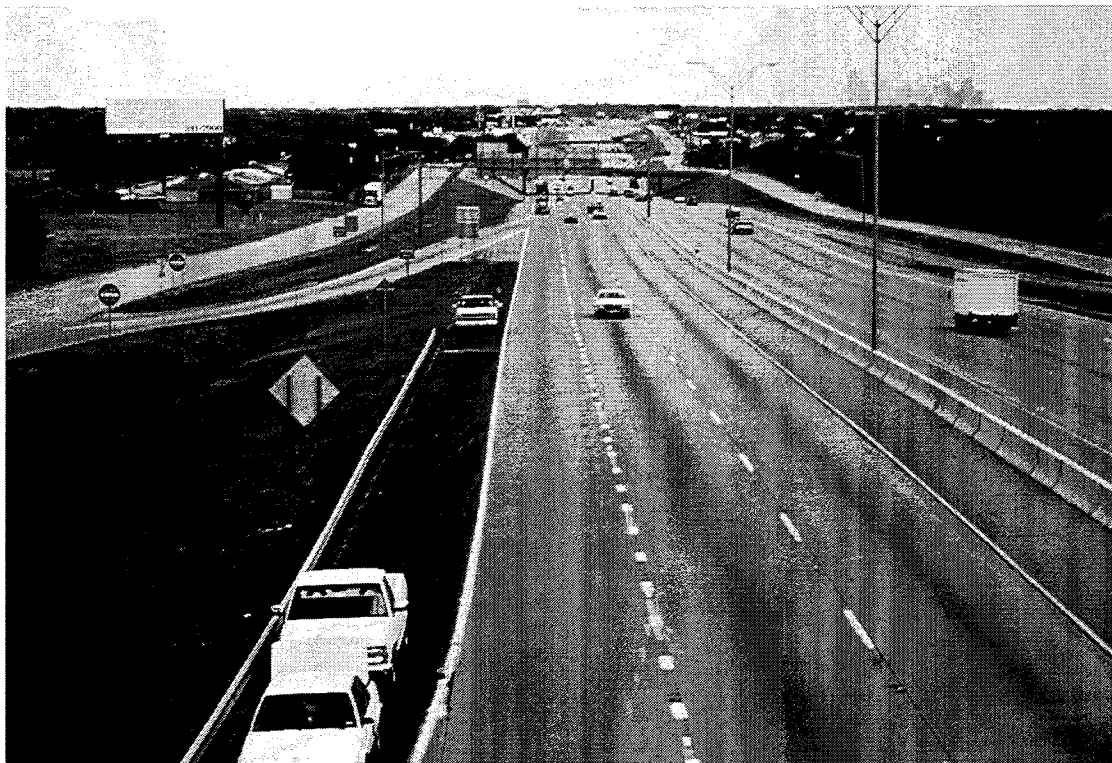
Figure 63. Lane Drop Markings at Site 7.
