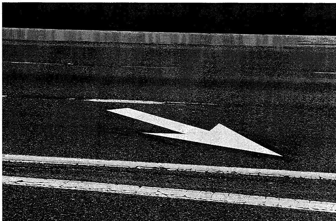
Figure 64. Pavement Arrow at Site 7.
