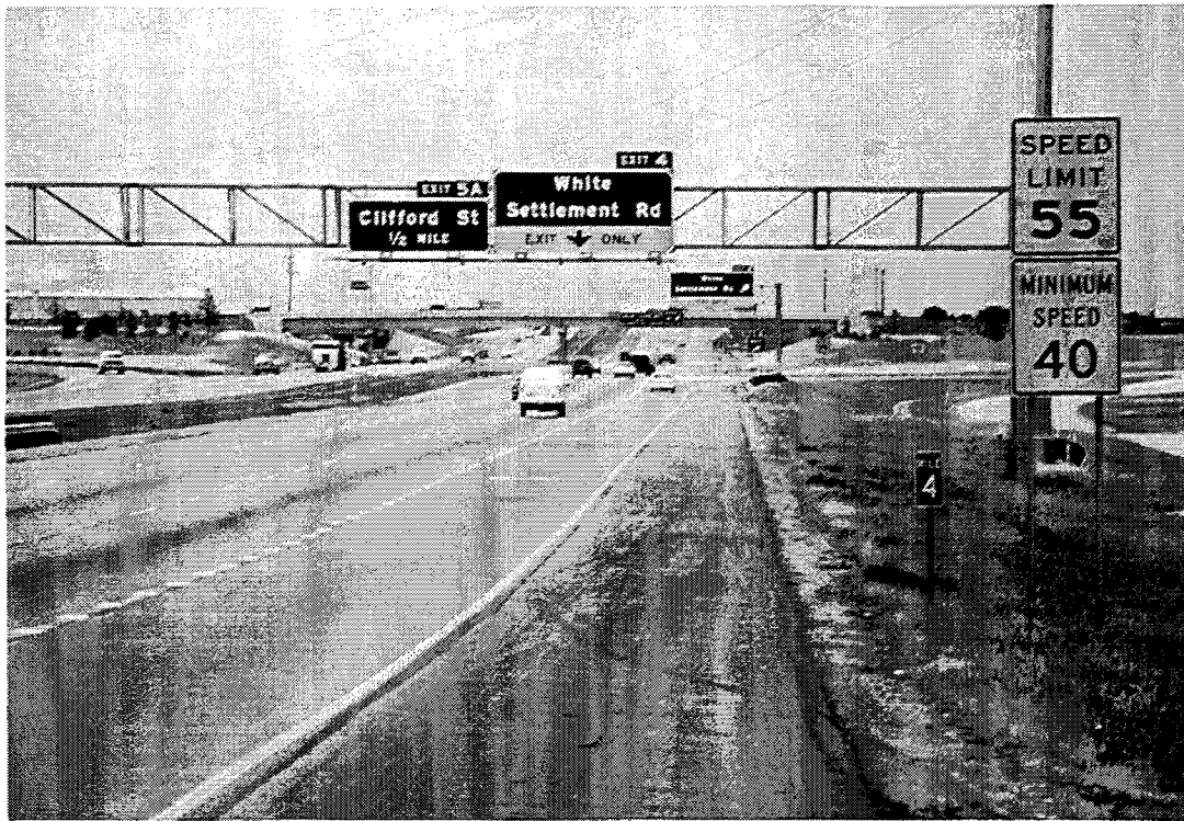
Figure 43. Lane Drop Markings at Site 3.
