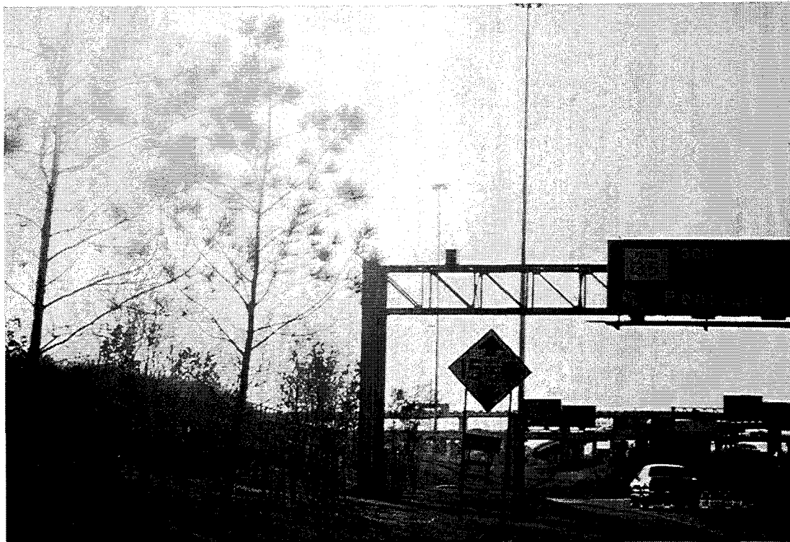
Figure 20. Mounted Camera on Sign Structure.
