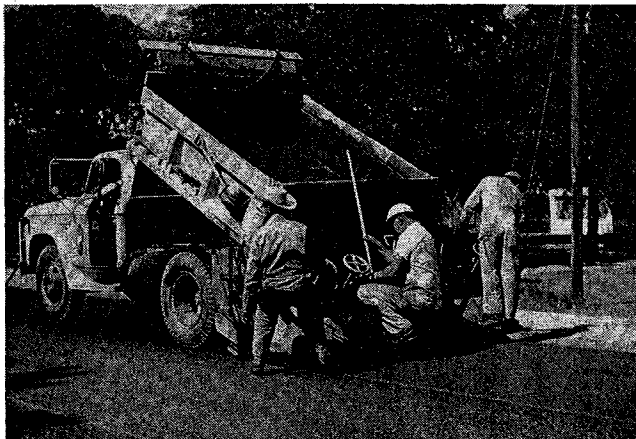
Figure 15. Use of the maintenance paver for the application of a cold mix overlay.
