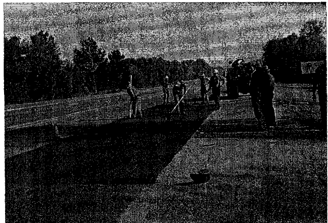
Figure 25. Hand raking cold mix for surface level-up.
