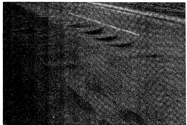
Figure 28. Typical example of transverse rutting (plastic instability).
