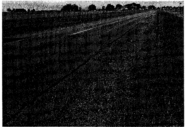
Figure 9. Typical example of edge raveling.
