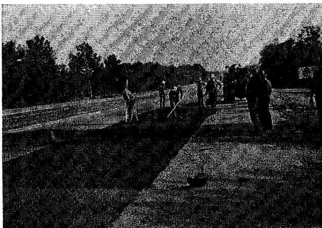
Figure 11. Hand raking hot mix-cold lay material for surface level-up.
