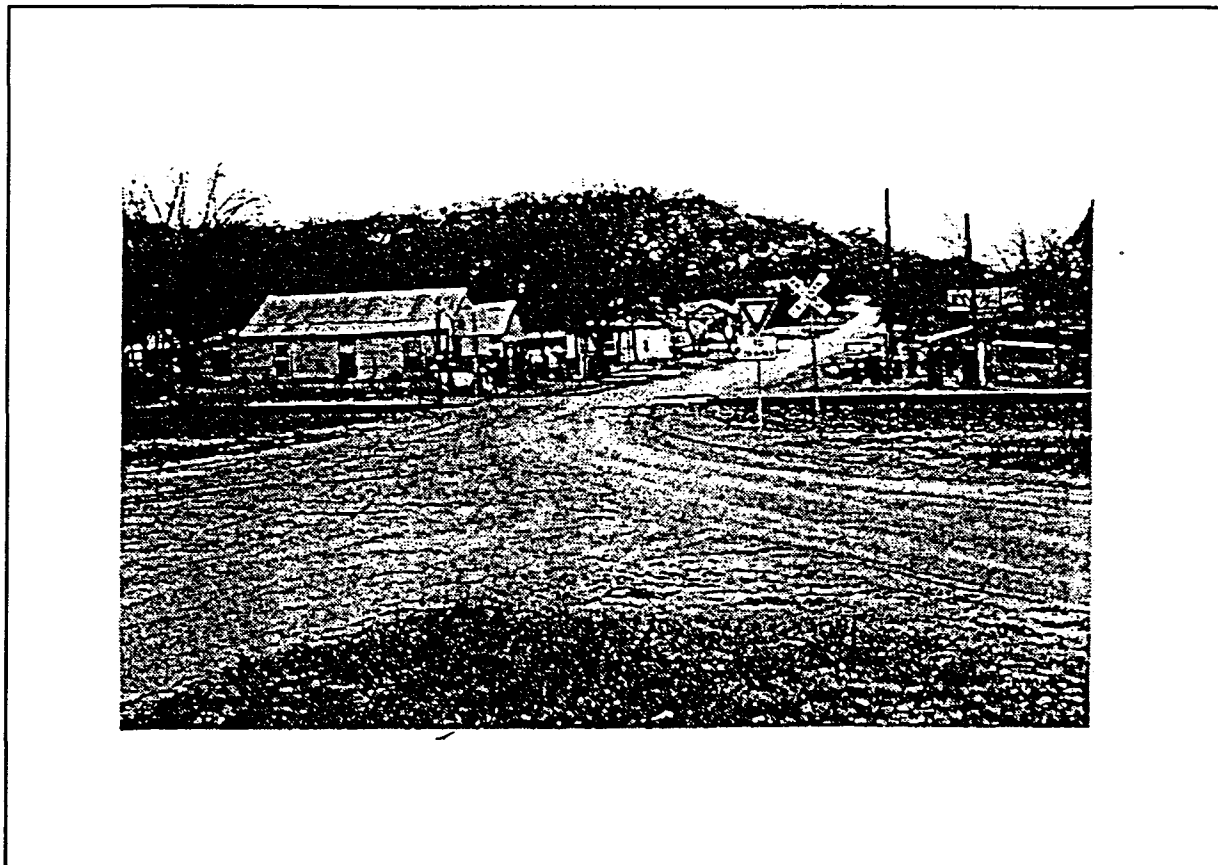
Figure I-3. Parker Street Crossing
