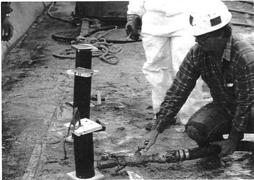
Figure 10. Field-grouted cable-stay specimens.
