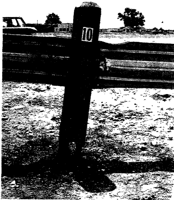
FIGURE F-51. Damage at Posts 9 and 10, Test 1263-3
