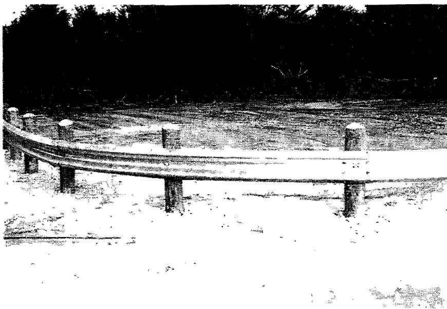
FIGURE V-5. Test Article Prior to Test 1263-2
