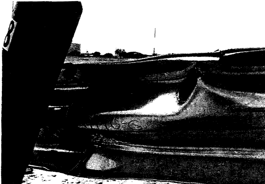
FIGURE F-49. Damage at Post 8, Test 1263-3
