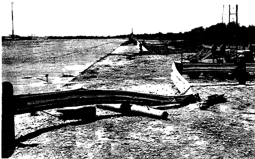
FIGURE F-11. Site after Test 1263-1
