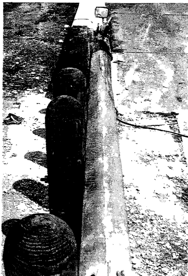
FIGURE F-66. Guardrail End Treatment after Test 1263-4
