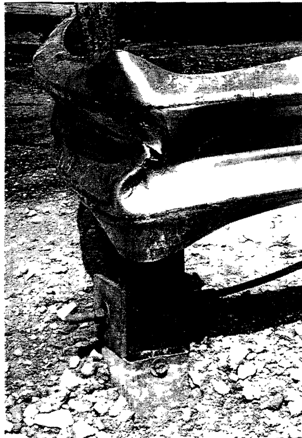
FIGURE F-50. Damage at Post 7, Test 1263-3
