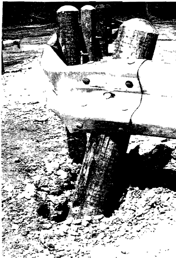
FIGURE F-31. Damage at Post 10, Test 1263-2
