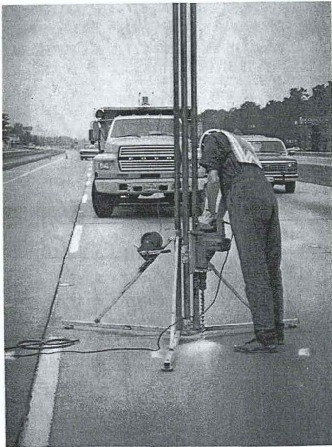
a) Drilling Dry Hole
