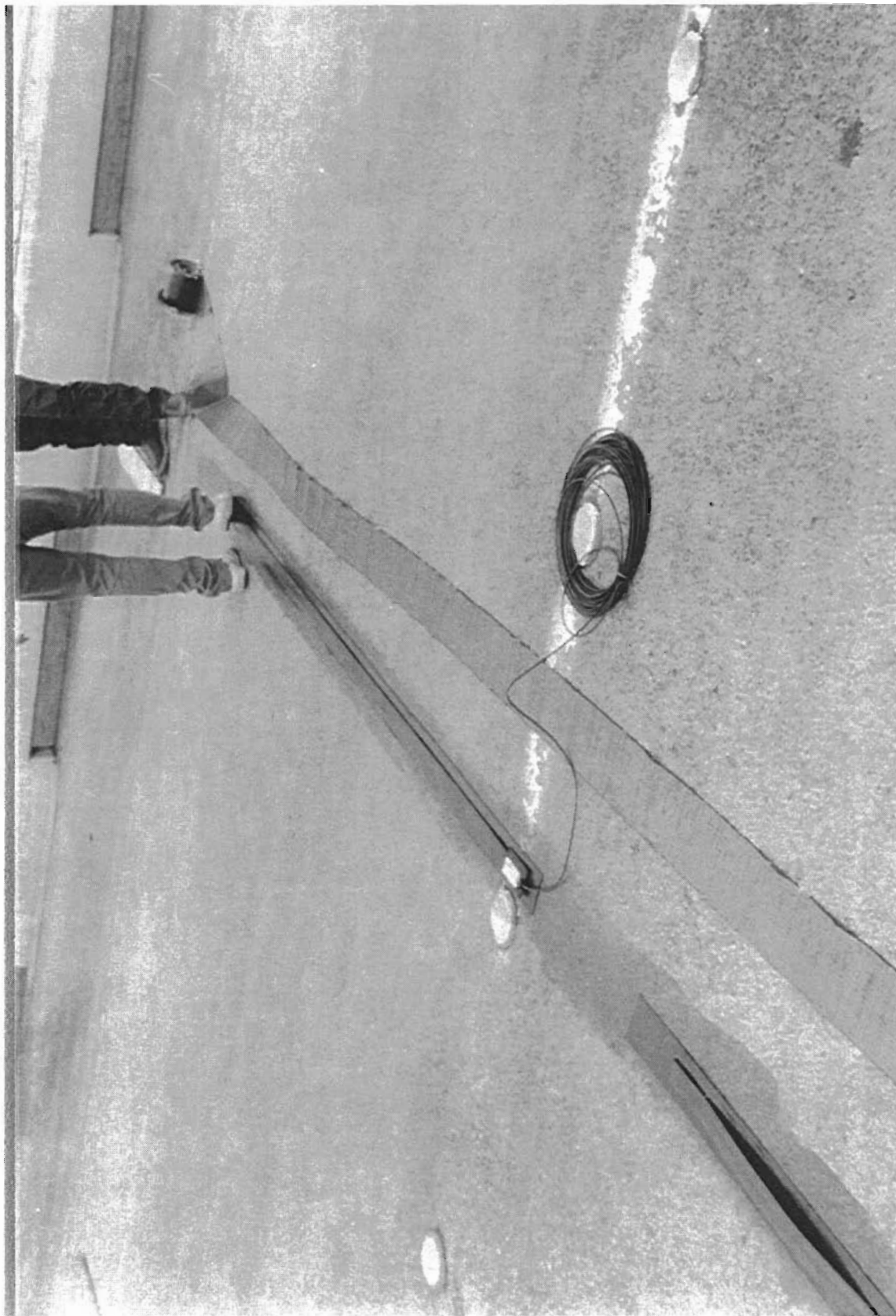
Figure 2-2. Lane 2 Piezo Sensor Prior to Covering with Polygard
