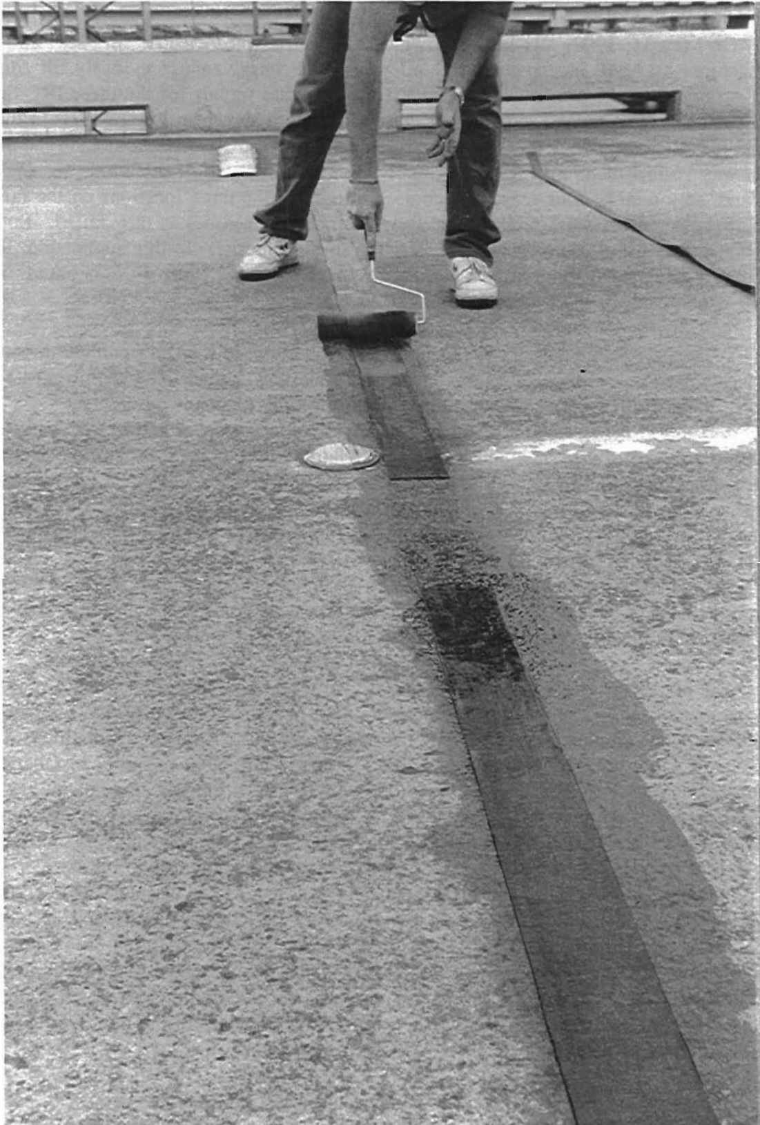
Figure 2-1. Applying Polygard and Primer for Piezo Sensors
