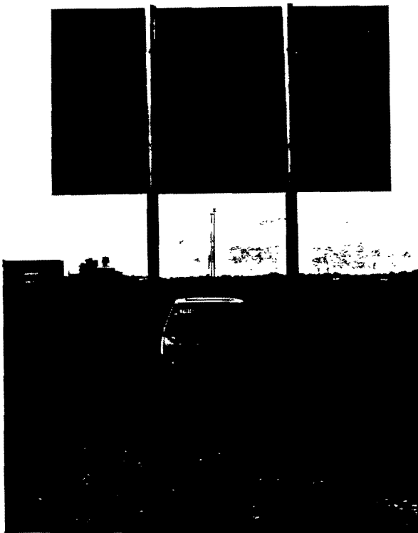
Figure 44. Sign installation before test 1219-6.
