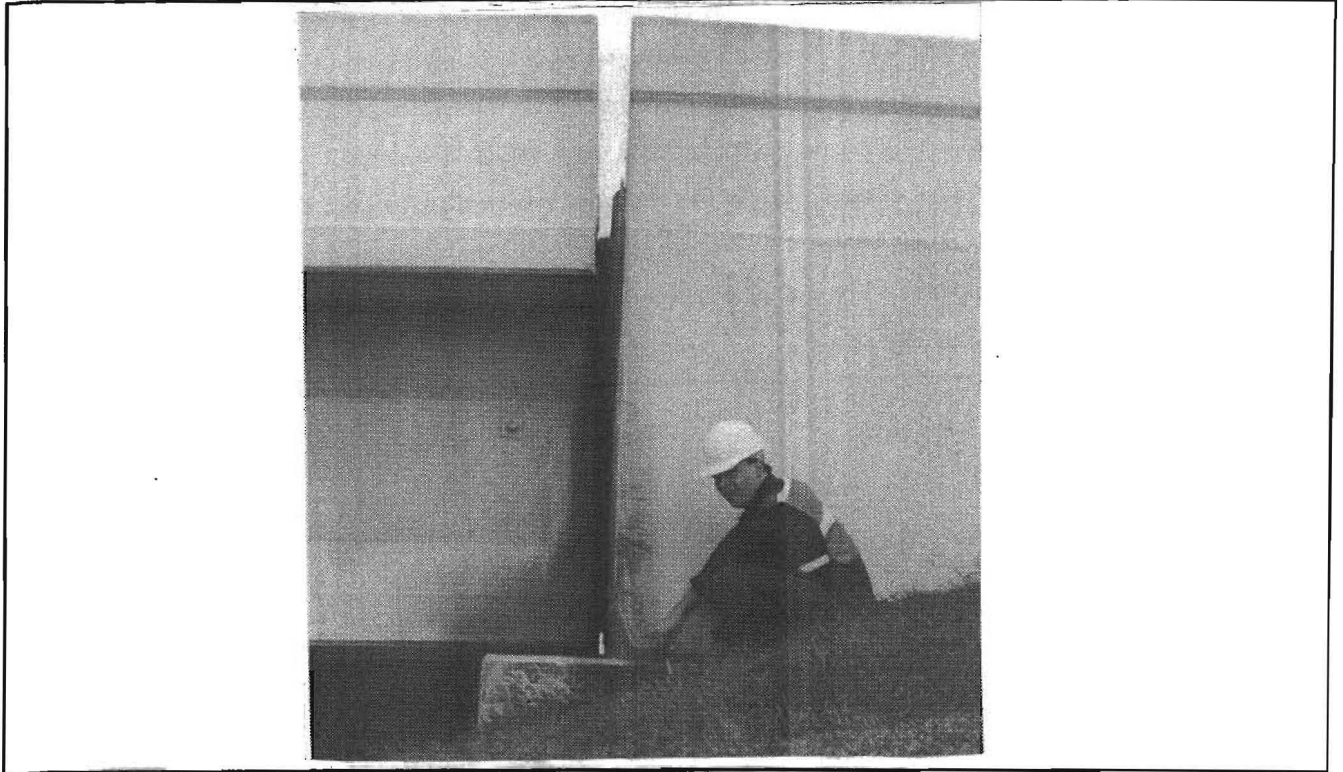
Figure 22.--Rotated Abutment and Wingwall (FM270 at Clear Cr. in Galveston Co.)
