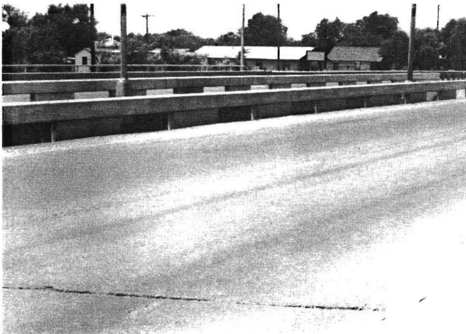
Photo # 5 -- Roadway Surface of Bridge Deck with Epoxy-coated Rebar
