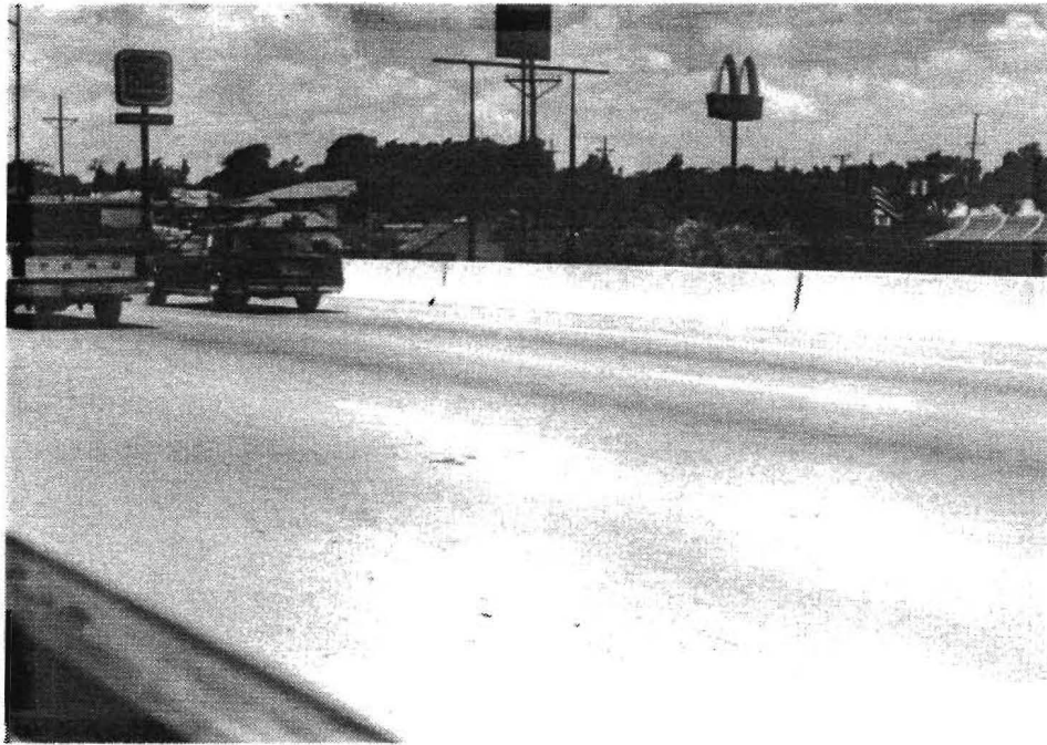
Photo # 7 -- Dense Concrete Overlays on Bridge Deck
