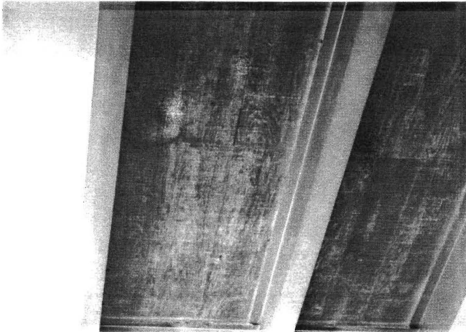
Photo # 4 -- Underside of Bridge Deck with Epoxy-coated Rebar
