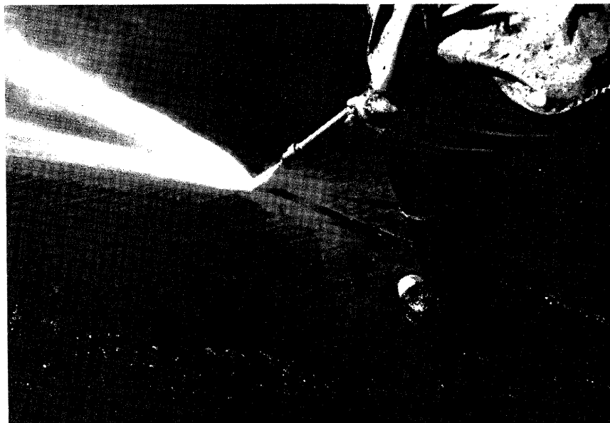
Fig. 2. The jet stream from the hand-held gun blew out the debris and seal materials in the top few inches of an expansion joint.
