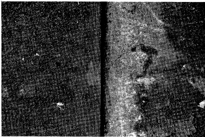
Fig. 16. Almost all detectable debris can be removed from fixed joints in pan-formed bridges.
