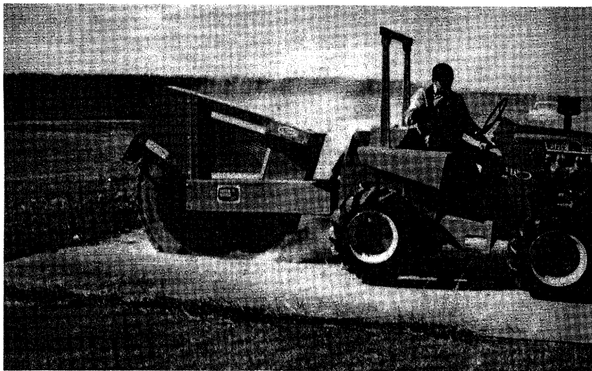
Figure 8: "Ditch-Witch" tractor mounted concrete cutting saw.
