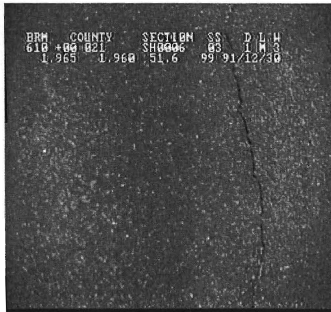
Figure 2. Longitudinal Cracking.
