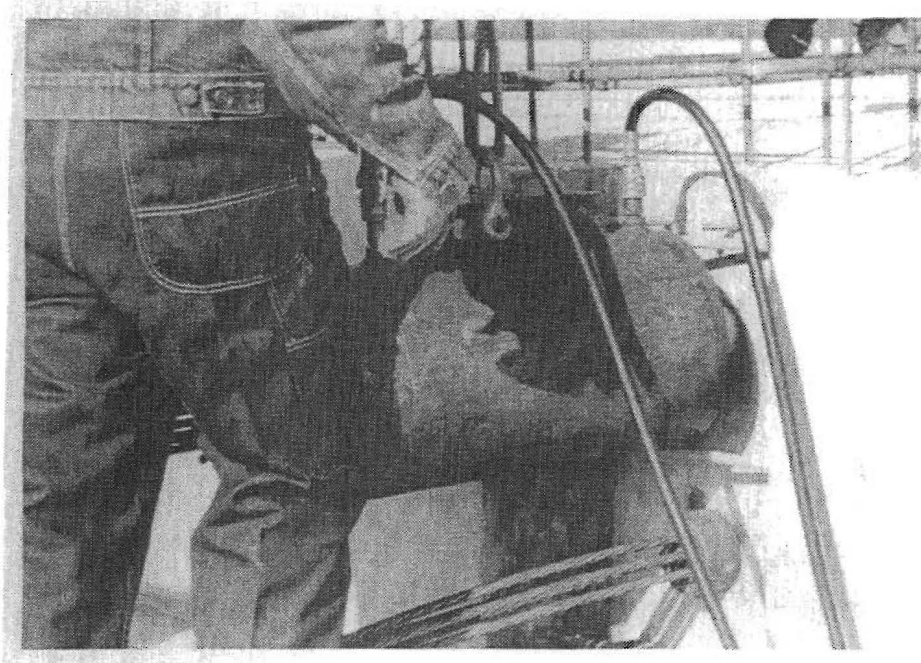
FIG. 18. Tendon Stressing Jack
