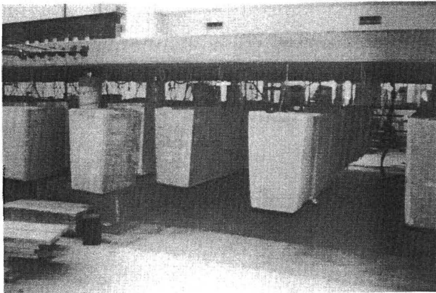
FIG. 15. Dead Weight Compensating Blocks are Suspended from Slab
