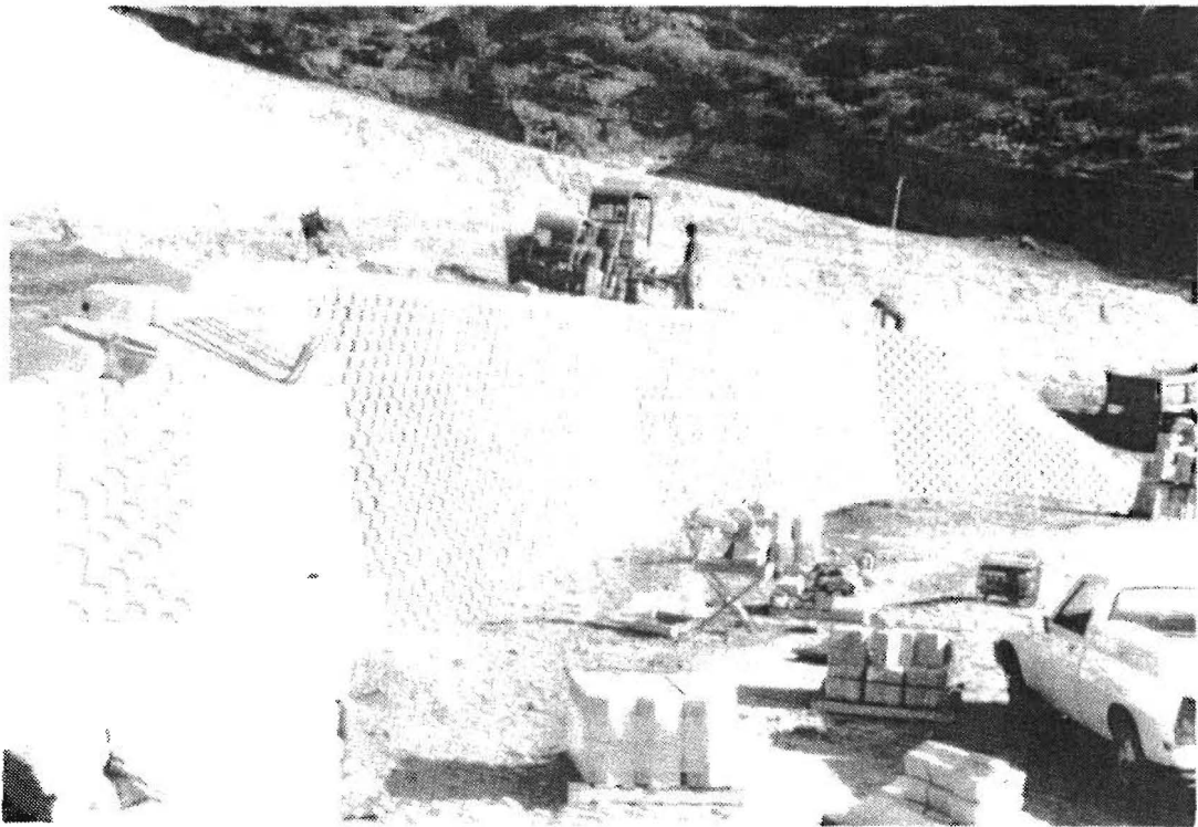
Figure 2.3 Compaction of cement stabilized fill
