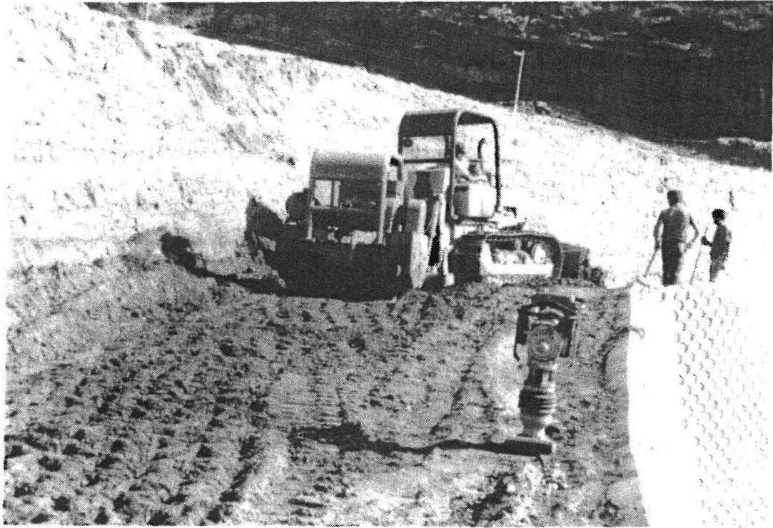
Figure 2.3 Compaction of cement stabilized fill
