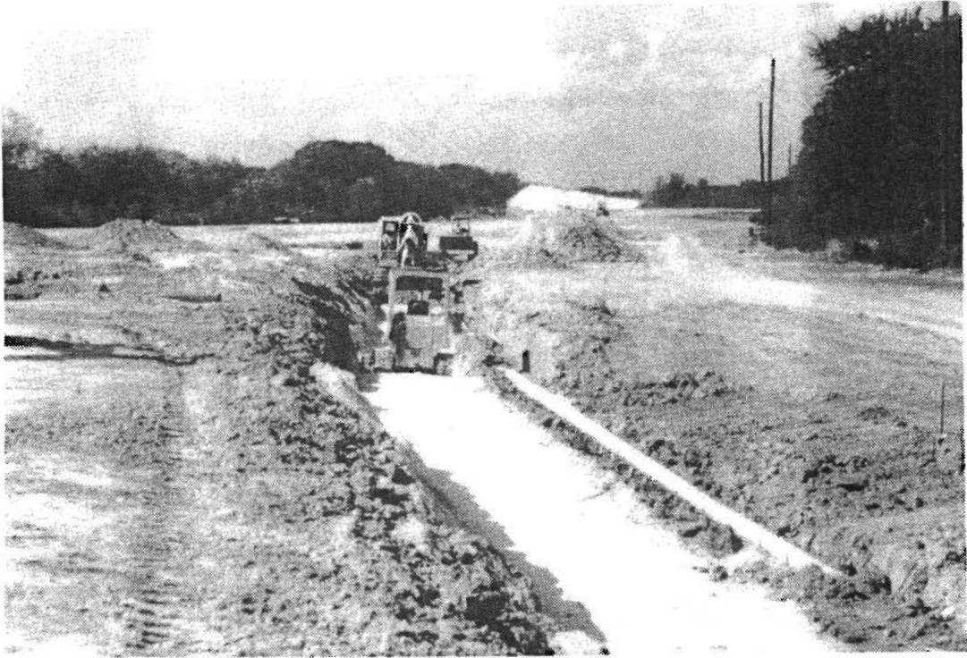
Figure 6.4 Foundation preparation for wall 7
