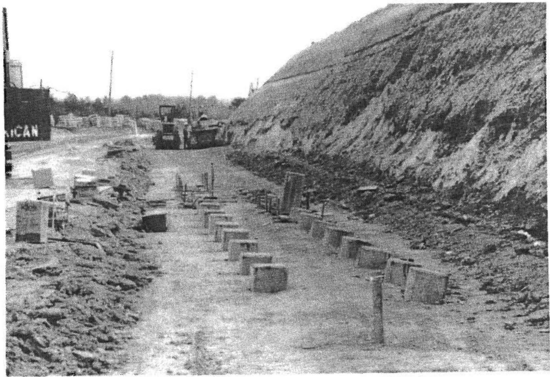
Figure 7.13 Photograph of piled foundation for wall 7
