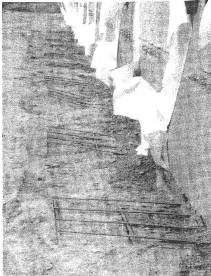
Figure 6.5 Facing panel anchors at wall 7
