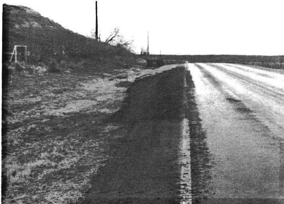
After patching with Brownwood Design
