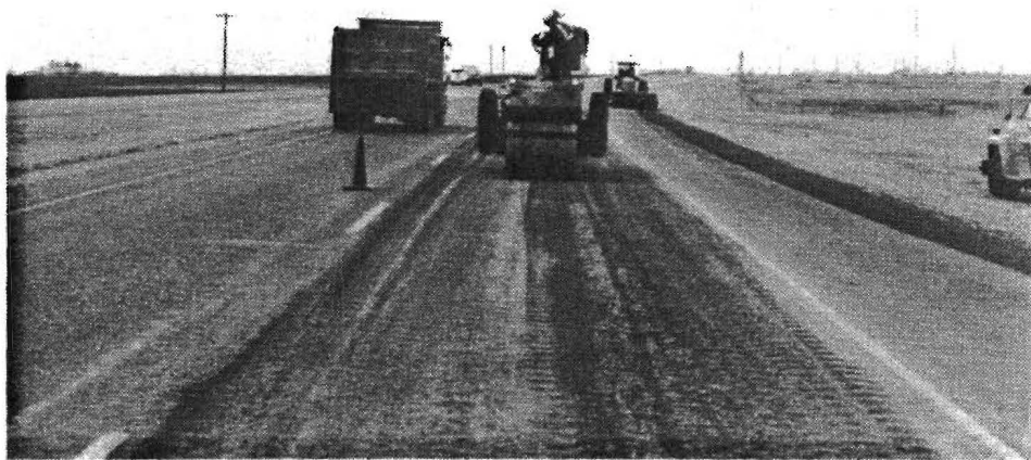
Blade-on application in progress
