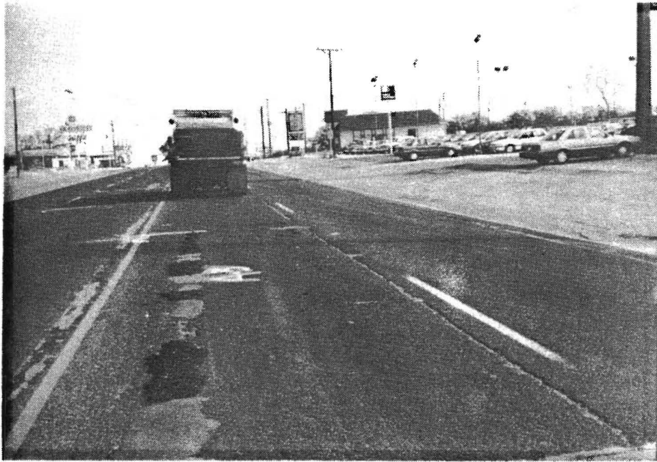
Potholes being repaired with New LRA
