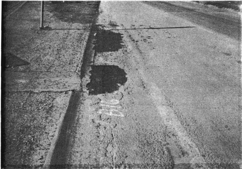
Compaction with truck tires
