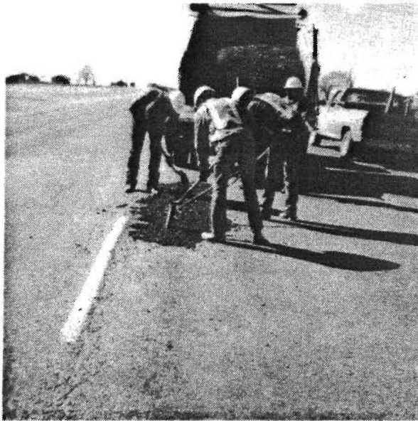
Pothole repair in progress with UPM
