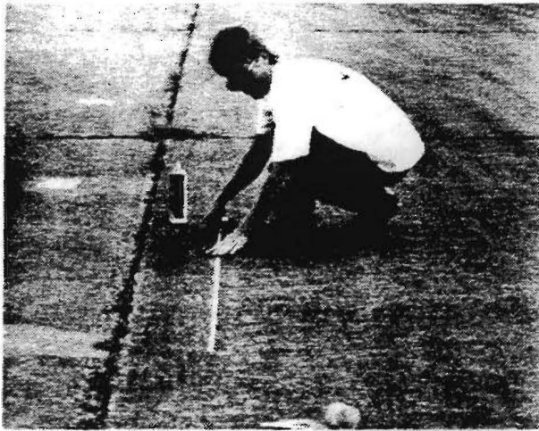
Figure 9.1 Temporary Loop Installation Photos (Continued)
