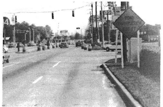
E. Field Placement of Advance Road Construction Sign
