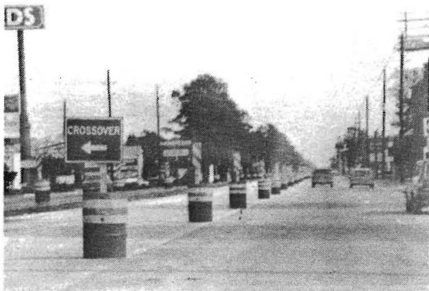
B. Field Placement of CROSSOVER Sign
