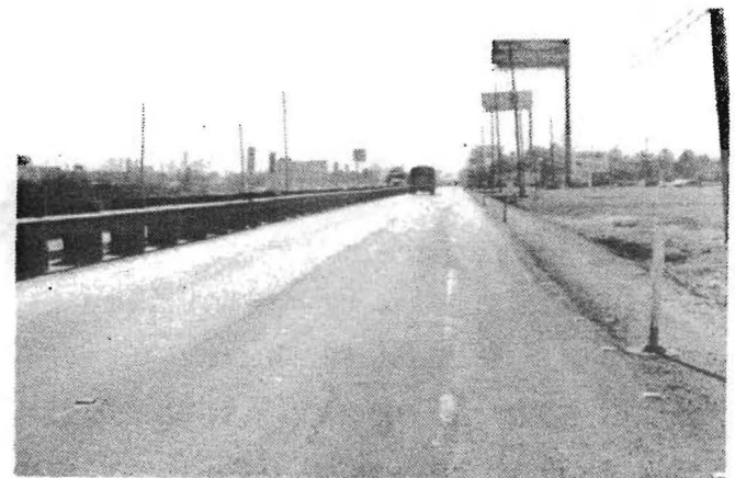
E. Field Placement of White Delineator Post
