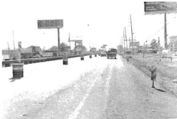
C. Field Placement of Vertical Panel
