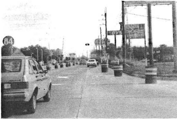
A. Field Placement of Chevron Panel
