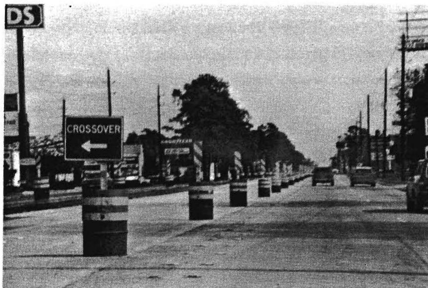
Figure D-23. Field Placement of Crossover Sign
