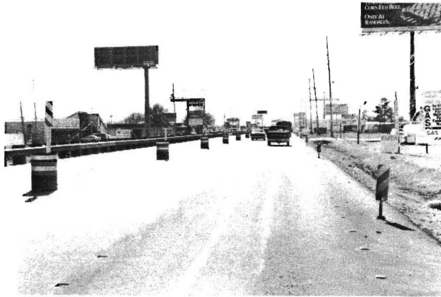
Figure D-14. Field Placement of Construction Object Markers
