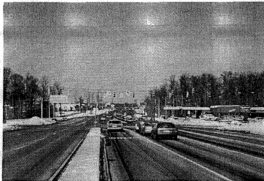
Figure 2-2. Depressed Single-Point Urban Interchange Located in Fairfax, Virginia.
