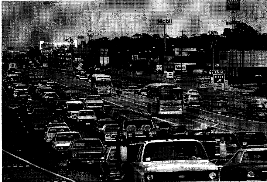
Figure 5. Transitway in Median of Katy Freeway
