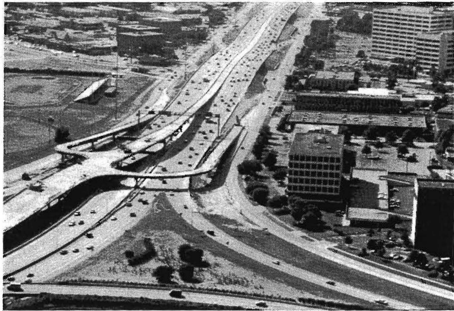
Transitway Ramps to Frontage Roads, Northwest Transitway
