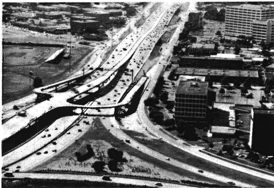
Transitway Ramps to Frontage Roads, Northwest Transitway
