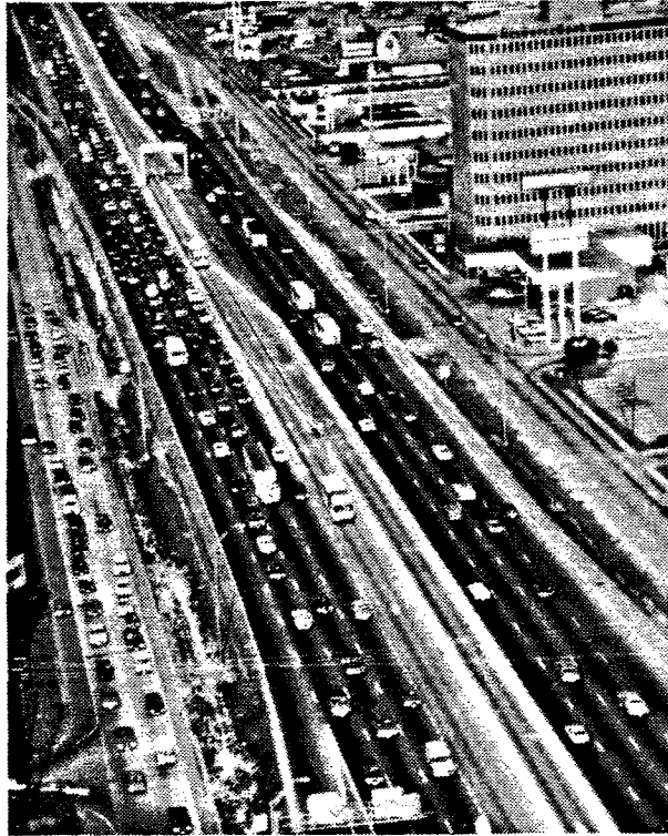
Figure 6. Slip Ramp for Transitway Access/Egress on Katy Freeway
