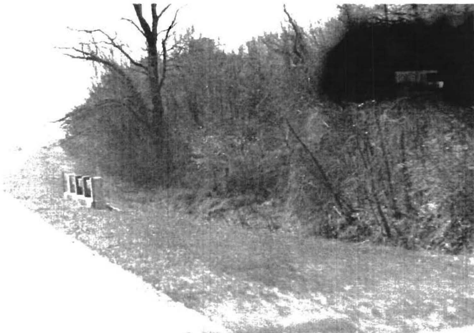
Figure 5: Concrete Rail Style Culvert Headwall
