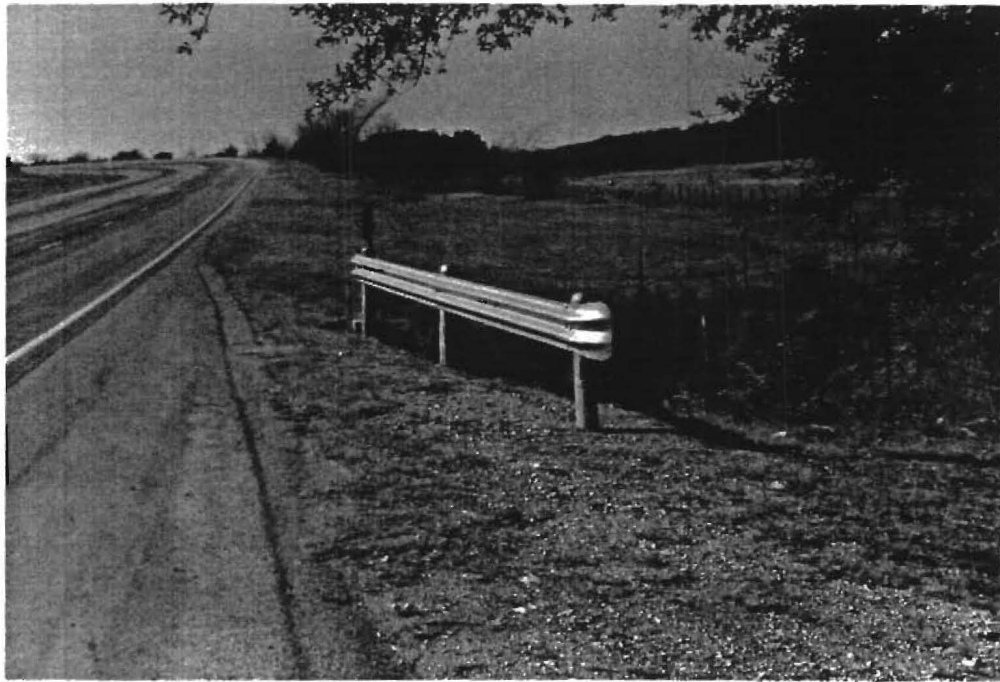
Figure 11: Short Segment of Rail in Advance of Drainage Structure
