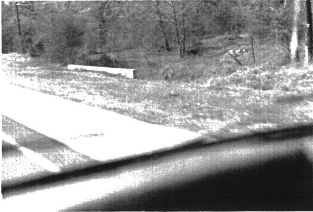
Figure 2: Drainage Culvert Headwall
