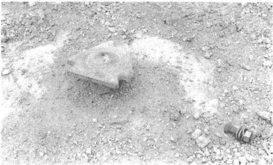
Figure 126. Sign installation after test 1122-11.
