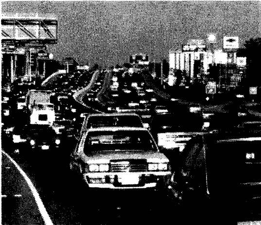
Figure 11. Katy Freeway and Transitway, Houston
