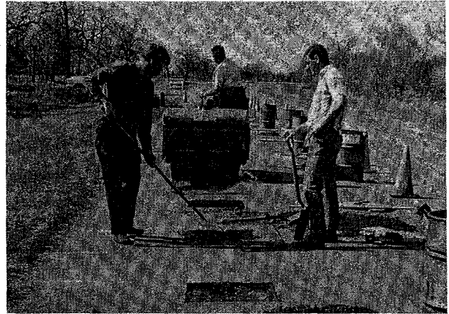
Figure 20. Field test plots of cold mix.
