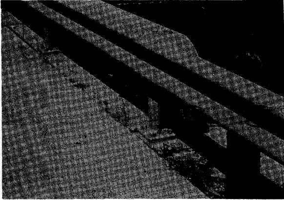
a. Full Beam Strength Developed Because Rail is Carried Across Bridge
