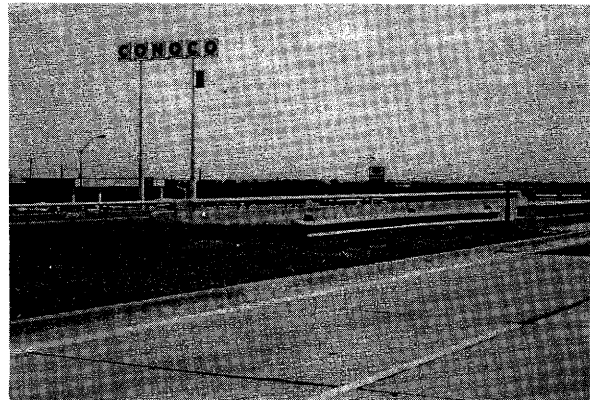
d. Open Gap Semi-protected by Short Guardrail Section. Vehicle can Easily Enter Gap (Code 12-01)
