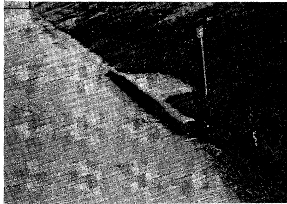
c. Curb Inlet (Inventoried as Non- Mountable Curb Less than 10 Inches High) (Code 05-02)
